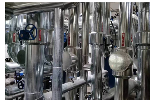
Replacement of heating valves
