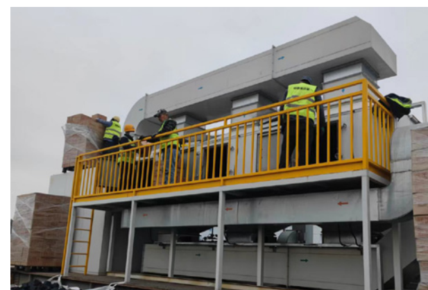
Replacement of activated carbon in two adsorption catalytic combustion units
