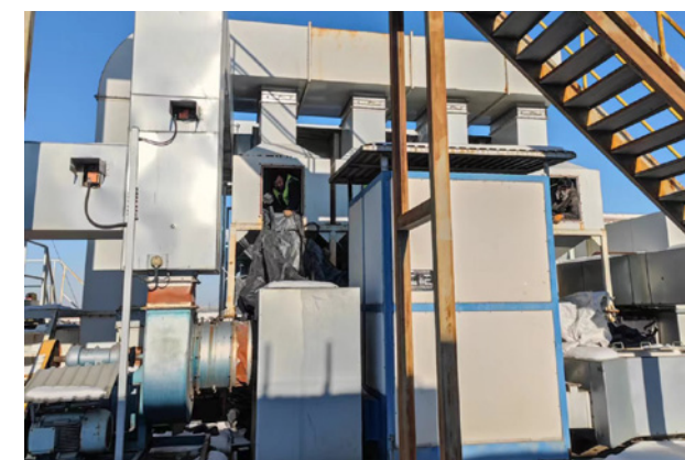
Replacement of activated carbon in two adsorption catalytic combustion units
