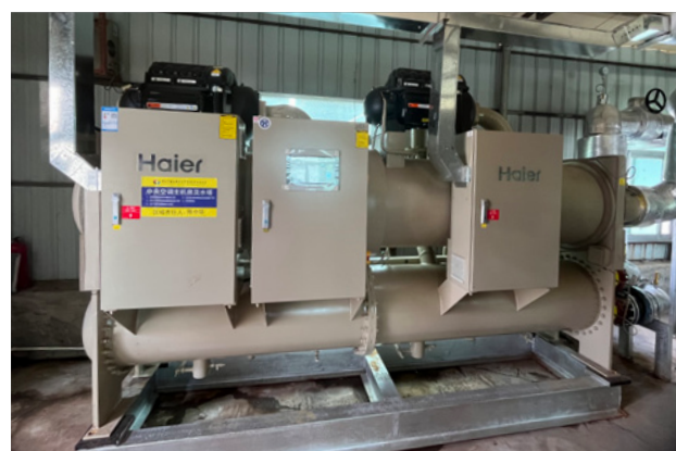
Replacement of cooling systems with magnetic levitation air conditioners
